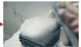
4. First layer coating
